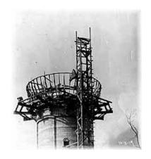
Just a skeleton version of the finished project, the water tower bowl begins to take shape. A worker appears precariously poised on the far right and a wooden open air elevator brings building supplies to the tower's final stages on Oct. 3, 1919.
