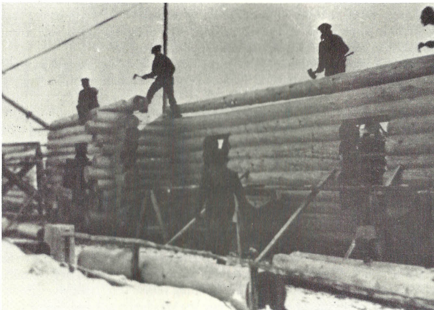
Construction of the Lodge, 1922-24.
